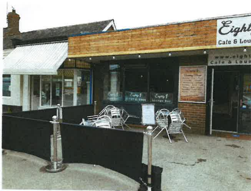
Figure 4 Left side of shop frontage
