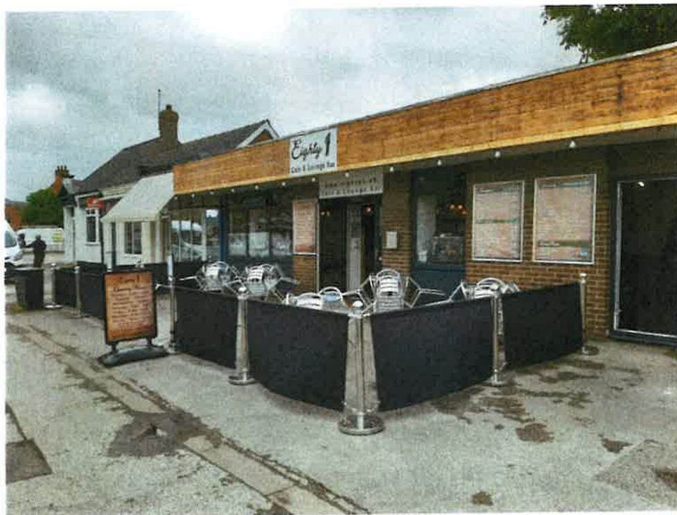
Figure 2 View from Level crossing
