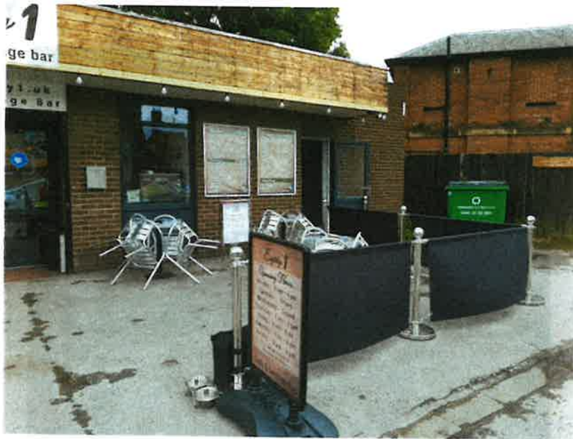
Figure 3 Right side of shop frontage
